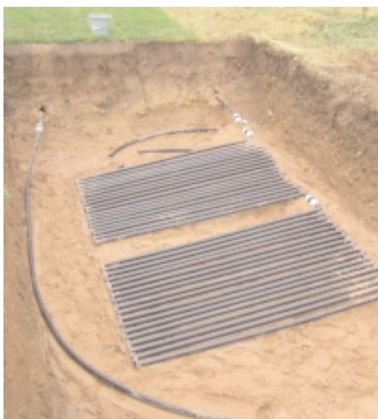
Saving energy: the 'Slinky' ground loop is buried 1m below the surface of the ground (top right); a £1500 grant is available for each domestic installation (bottom right); compact collectors are used where garden space is limited (bottom left); 'Ice Energy Greenline Heat Pump' (above)
